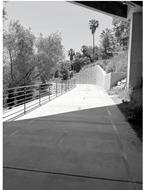
This view of the newly opened Dry Creek Trail, Phase 1, is where the trail emerges from under I-80.
